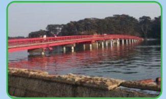
Fukuura Bridge (Matsushima) repaired with donations from Taiwan
