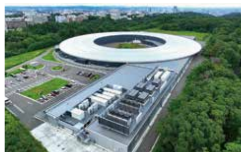
NanoTerasu, a state-of-the-art 3 GeV synchrotron radiation facility
