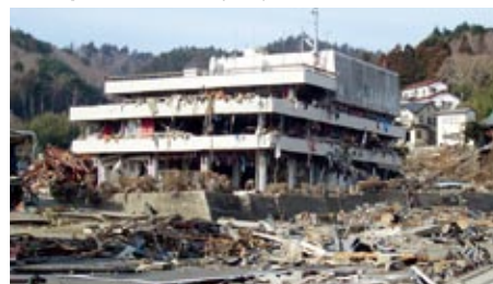
Onagawa Town (Government Office Building flooded to third floor)
