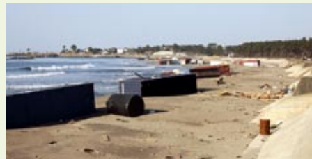
Shichigahama Town (Shobuda Beach littered with containers)
