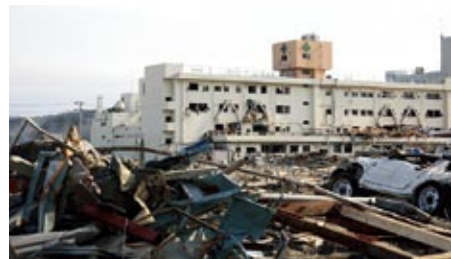
Minamisanriku Town (massive amounts of debris in urban district around Shizugawa Public Hospital)
