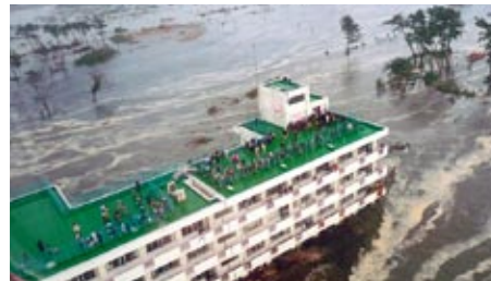
Sendai City (stranded Arahama Elementary School)
