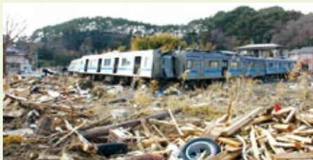
Higashimatsushima City (vehicles on the Senseki Line washed away by the tsunami)
