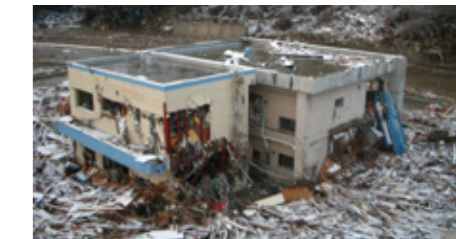
Photo: Wrecked fire department building surrounded by debris (Minamisanriku Town)
