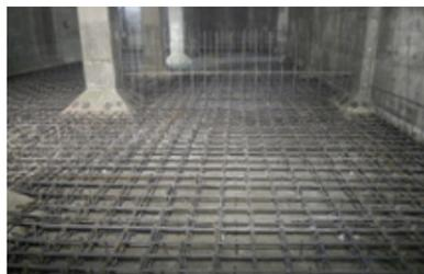
Photo: Fumotoyama No.1 regulating reservoir under seismic retrofit work
