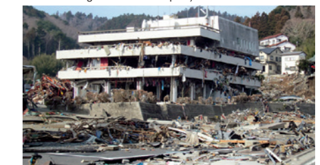
Photo: Onagawa Town (government office building flooded to third floor)
